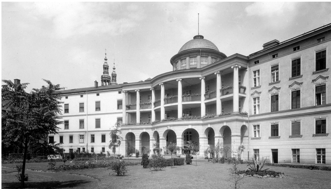
The Transfiguration Hospital in Poznan: view from the garden
